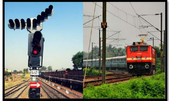
Colour Light Signals Located Outside All Tracks
